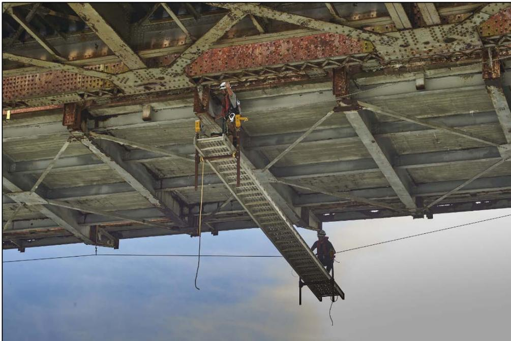
**Figure 4:** Below-deck inspection of truss from a pickboard
