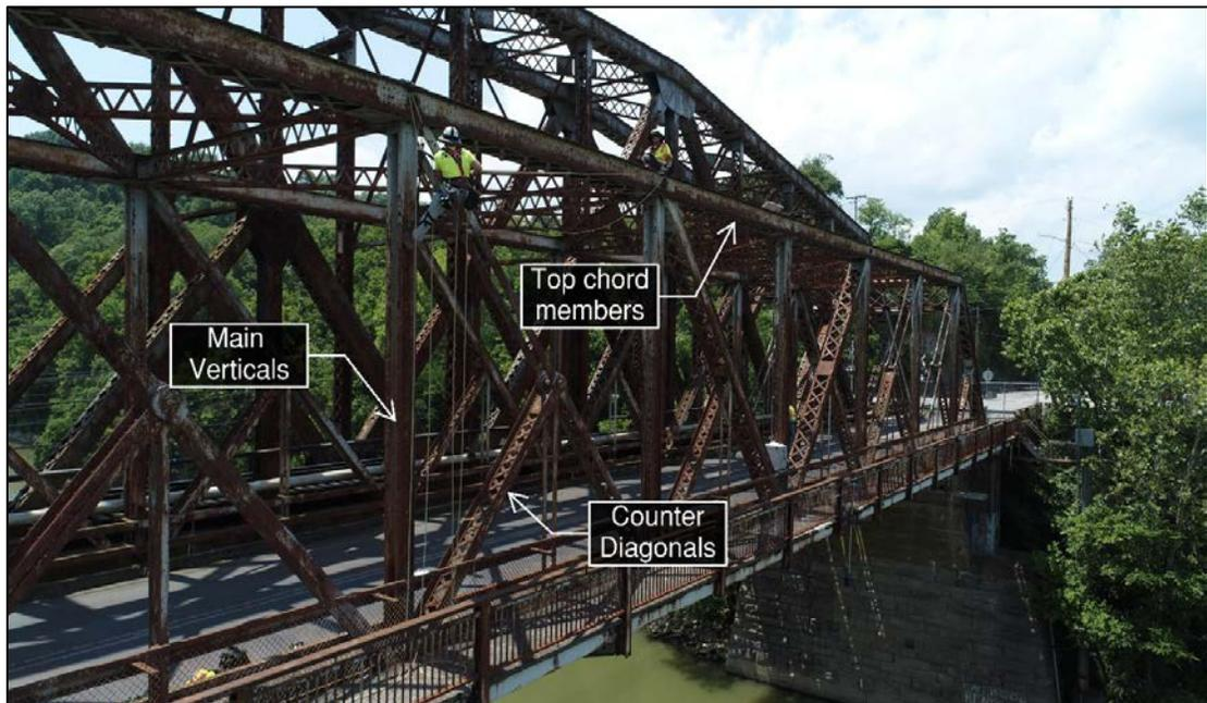
**Figure 9:** Truss member types above deck
