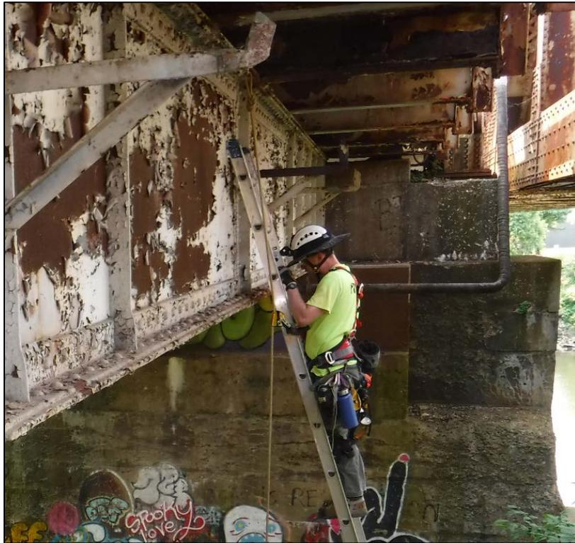
**Figure 5:** Girder inspection from extension ladder
