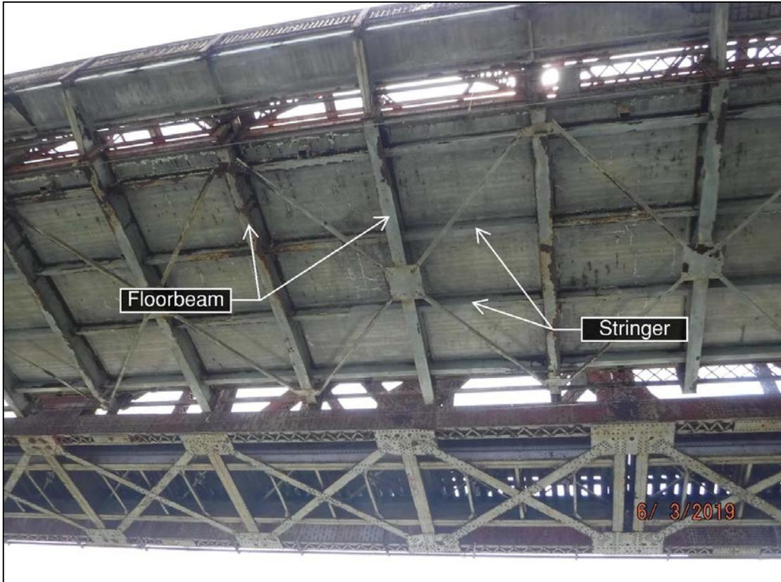
**Figure 8:** Truss member types below deck
