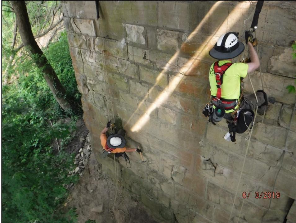
**Figure 3:** Inspection of pier using rope access in accordance with SPRAT
